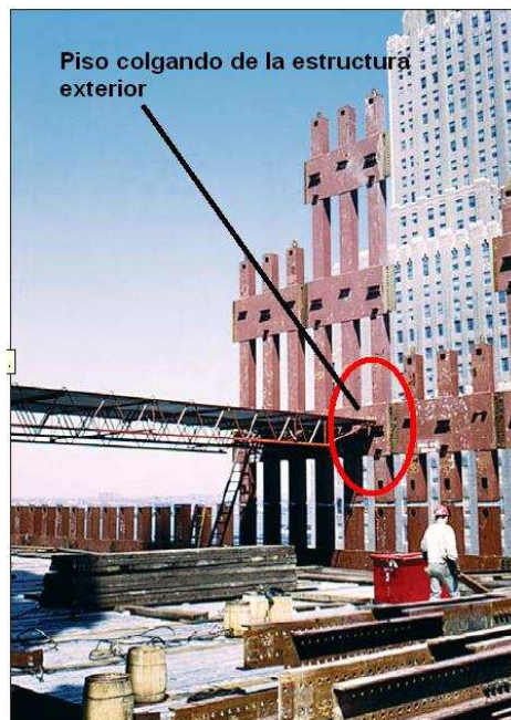
Figure 2-8 Erection of floor framing during original construction.
